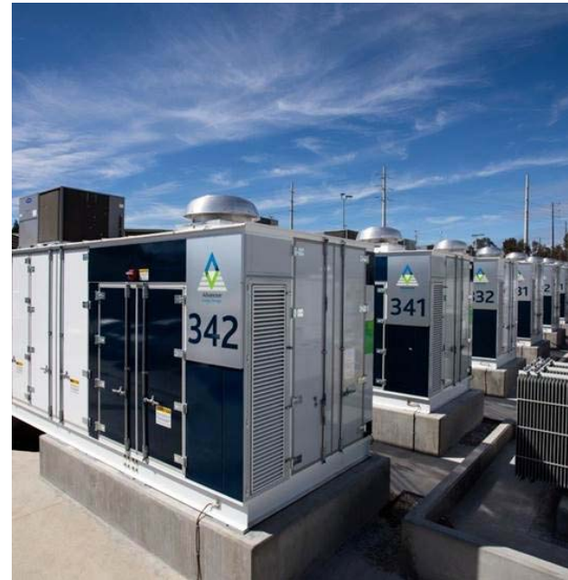
Caption: SDG&E's 30 MW / 120 MWh battery storage project in Escondido, largest lithium-ion battery system in the world
